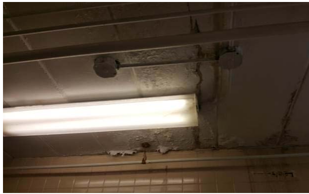
The image to the left is of the water damaged ceiling in the men's bathroom. And the image to the right shows flooding in the locker room during a storm event.
