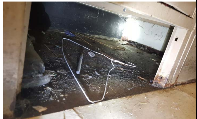
Left: View of the locker room ceiling showing water seepage. The ceiling tiles were replaced recently but the ongoing issue with water seepage and the resulting damage is evident. The image to the right illustrates the water damage under the lockers.
