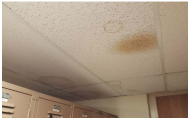
Left: View of the locker room ceiling showing water seepage. The ceiling tiles were replaced recently but the ongoing issue with water seepage and the resulting damage is evident. The image to the right illustrates the water damage under the lockers.
