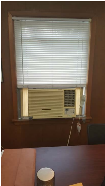
Wood panelled office space, which was originally a sunroom. Lack of insulation, inefficient heating and airconditioning requiring window units to be fitted during summer months and portable heaters during winter months.
