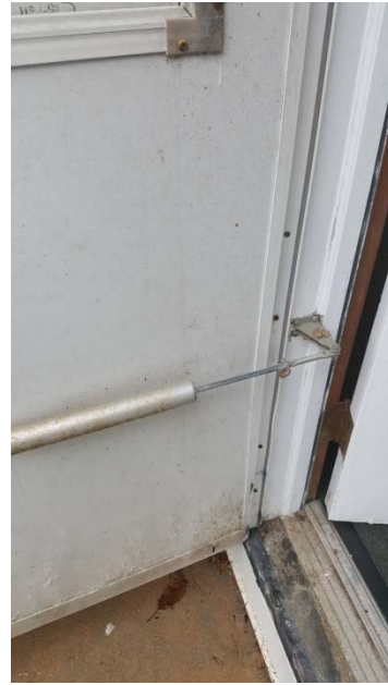
Storm door at the emergency exit located to the north of the building showing water damage.
