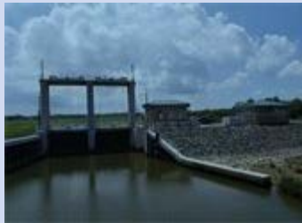
Pictured above is the new flood gate and pump operation at the Port Monmouth Flood Risk Management Project. Photo credit to U.S. Army Corps of Engineers and caption credit to Civil Structure + Engineer magazine.
