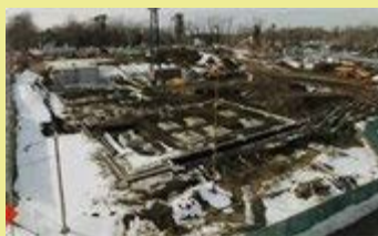
Town Hall construction on 2/17/21.
