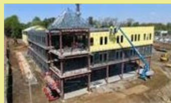
Town Hall construction on 5/11/21.
