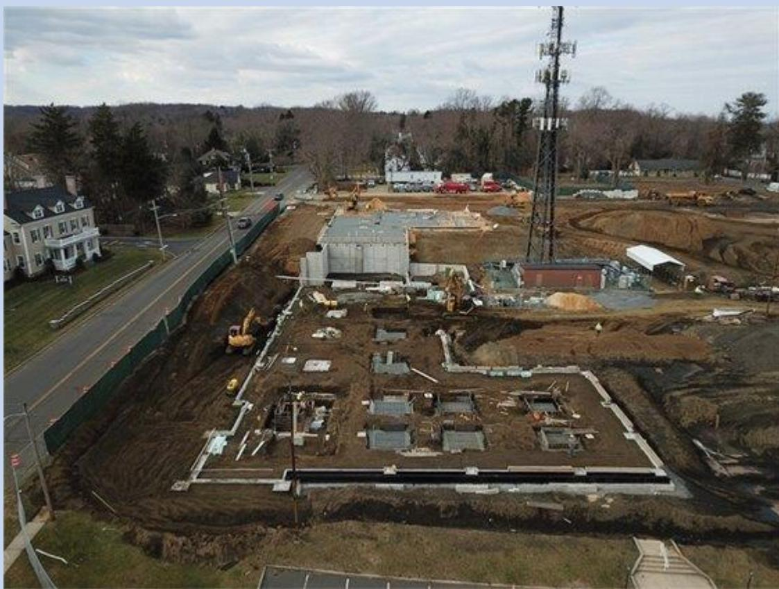
As of this week, the foundation and underground utility work at the new Town Hall (located behind the Police Station) is nearing completion. Site work around the building continues, including grading and storm water management piping. Underground plumbing and electric is also in progress. The slab floors are the next item scheduled to be completed, weather permitting. The next major phase will be delivery of a crane and
