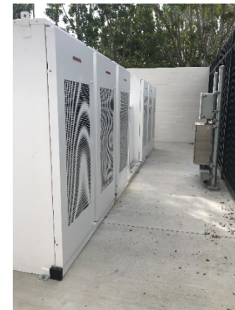
Typical <1MW Storage Unit
