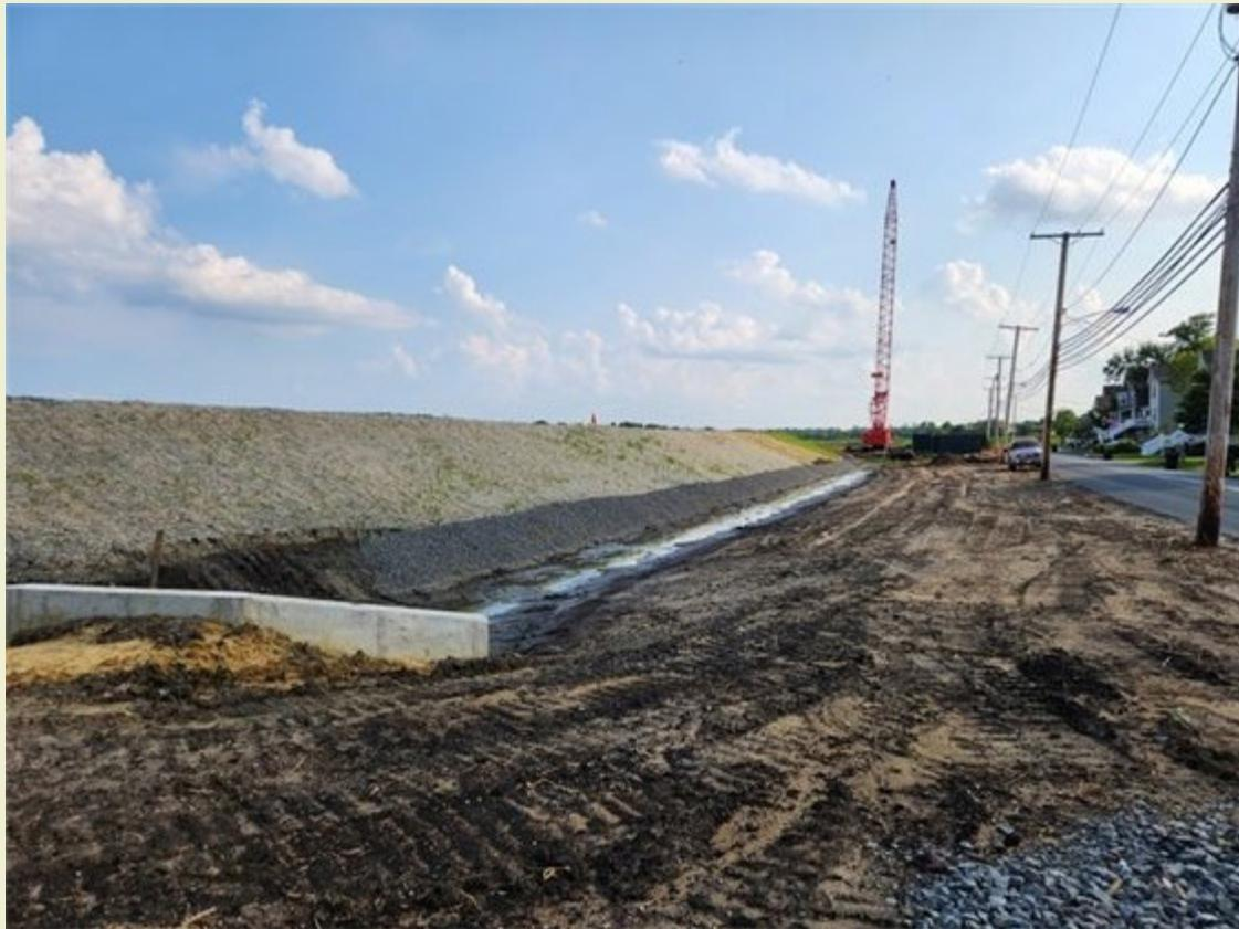
The U.S. Army Corps of Engineers' (USACE) Port Monmouth Flood Control Project continues along Main Street. The current phase of the project includes pile driving for a floodwall that will run from the recently built levee to a new road closure gate at Broadway.
