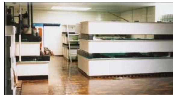
Figure 5.9: Self supporting stacked tanks, Source: Marine Biotech
