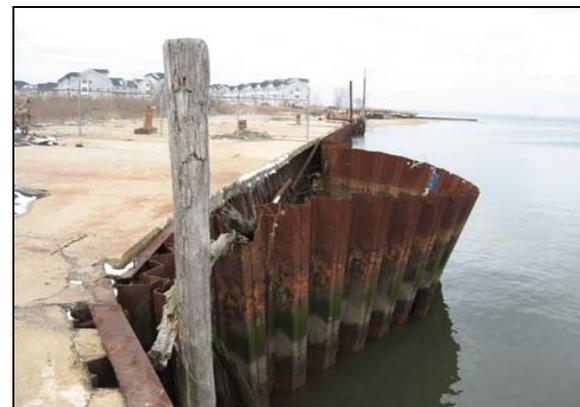
Figure 3.5: Deteriorating bulkhead
