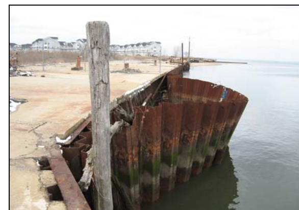
Figure 3.5: Deteriorating bulkhead
