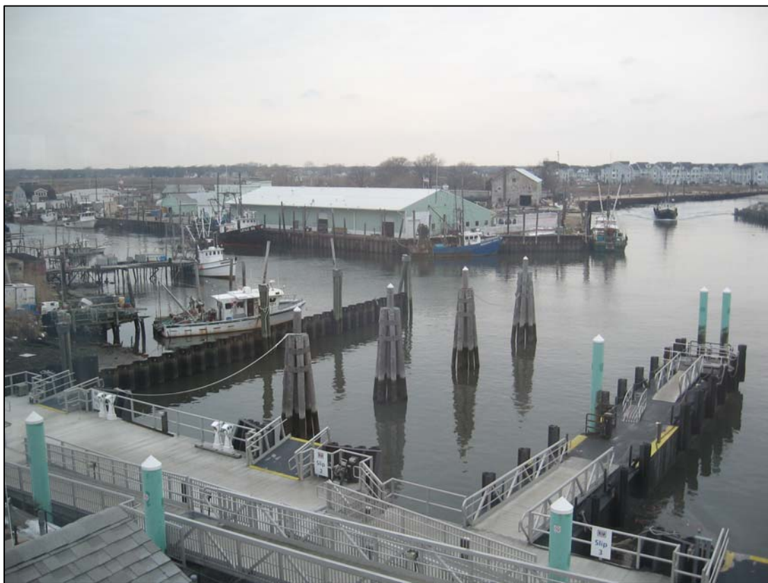
Figure 2.1: Study Area showing Parcel A and B. Figure 2.2: View from ferry terminal.
