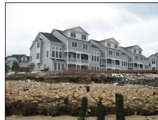
Figure 3.2: Adjacent residential development
